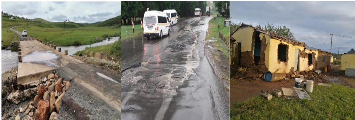
FIGURE 5: Floods Affected Bridges and Roads in 2022 (Source: HGD Disaster Management, 2022)
